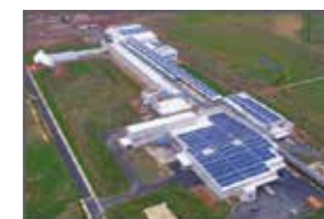
Rooftop Solar Power Plants • DG-PV Hybrid • Solar With Battery Storage
